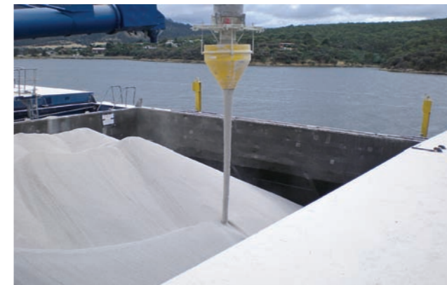
After installation of DSH System
